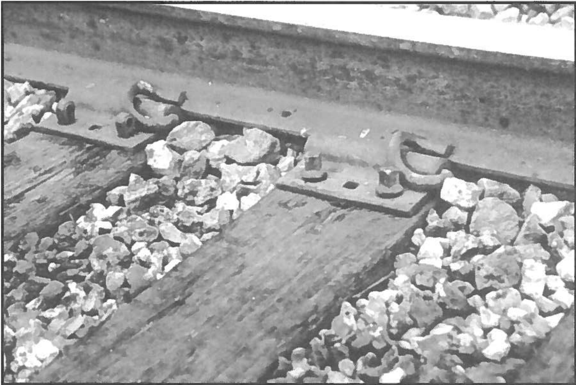
Photo 15: Parallam Ties with Pandrol plates & Clips (left with lock spike, right with screw spike)
