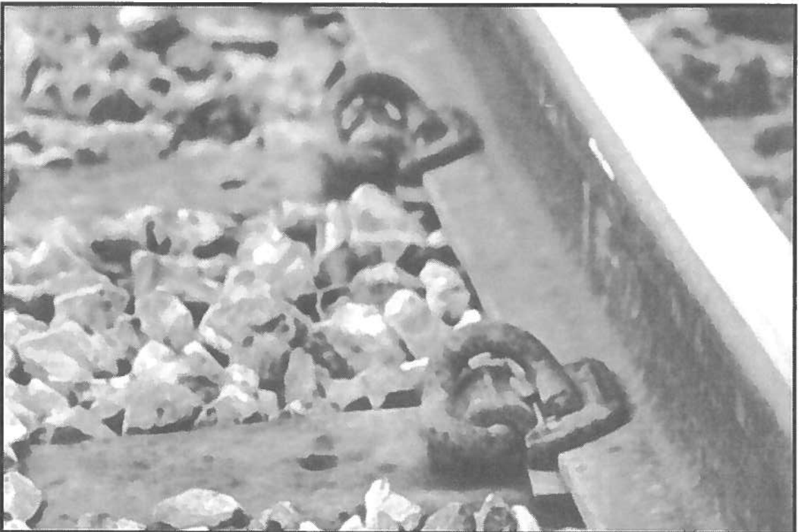
Photo 18: One of several steel tie designs
