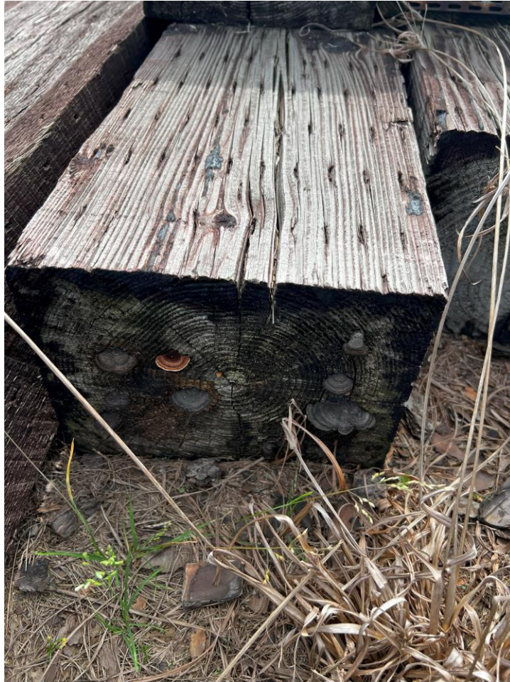
Figure 4 – Previously cut Douglas Fir tie with decay fruiting bodies.
